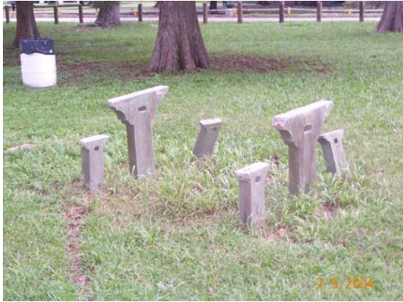
Figure 37. Deduct even more points for missing parts, as this limits the functionality of the picnic table.
