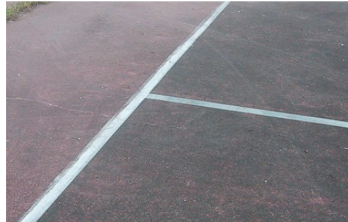
Figure 66. Example of painted markings on court that are clearly visible (1).
