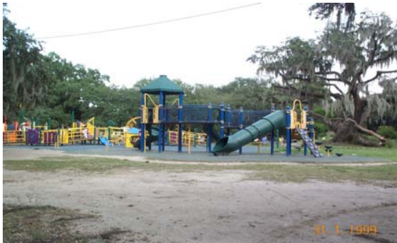
Figure 86. Example of "Unitary Synthetic Surface" (4) surrounded by turf (dirt). Assess only the surface that is directly underneath the play equipment. (Mark (4) only.)
