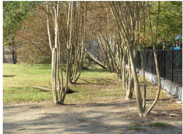
Figure 6. Evidence of tree & landscaping damage (note angle of trees in background)
