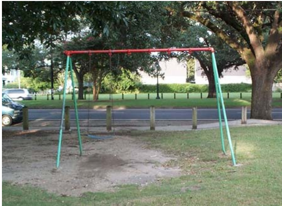
Figure 92. Example of missing swing.
