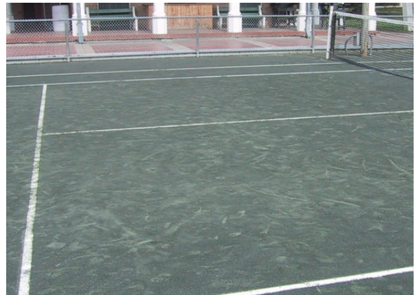
Figure 64. Deduct points for scuff marks that haven't been swept (specific to this particular surface type).
