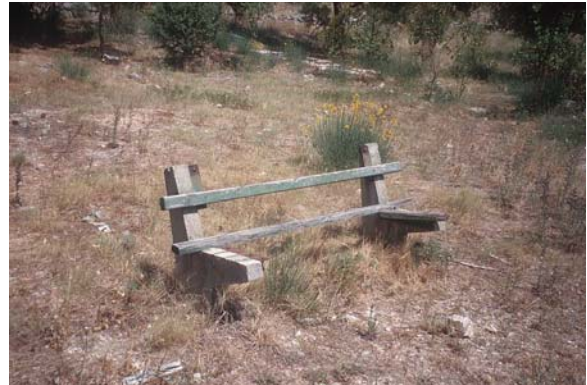
Figure 23. Even more points should be deducted for missing pieces, as this limits the functionality of the bench.
