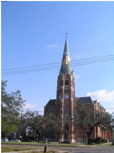
Figure 11. Wind damage to neighborhood buildings
