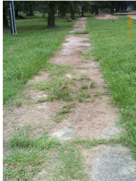
Figure 52. Example of a sidewalk. Points deducted for trip hazards and overgrowth.
