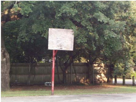
Figure 67. Deduct points for missing basketball hoops (making court unusable for playing basketball).
